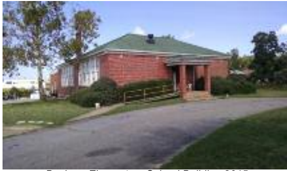
Buckner Elementary School Building 2015
